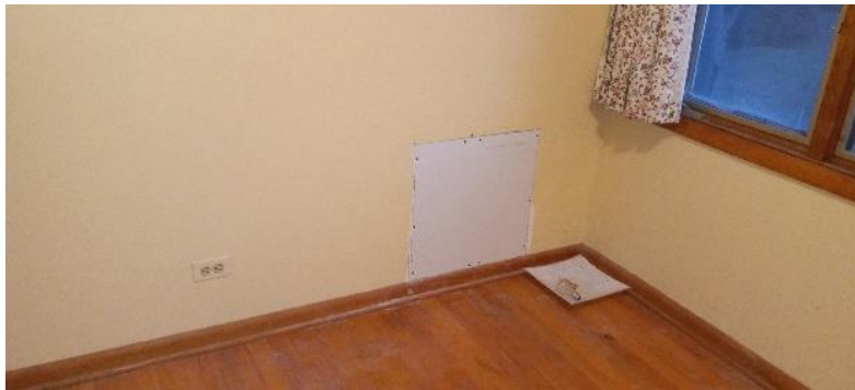
Paint walls upstairs
