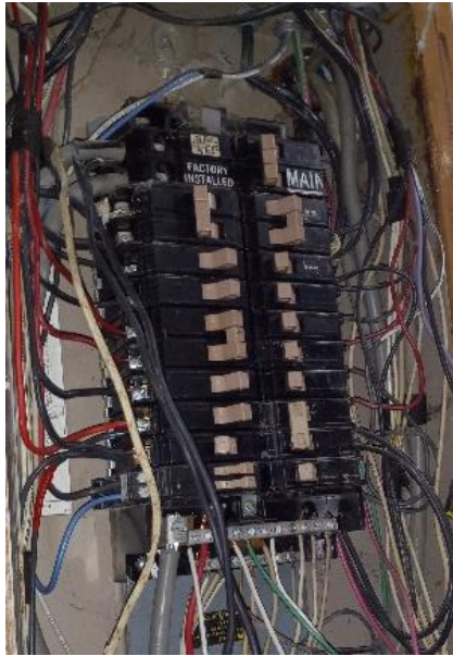
Replace Electric box and replace outlets in basement
