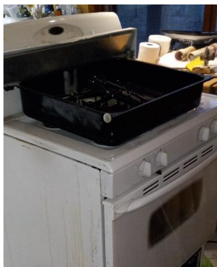
Install Kitchen Gas Stove
