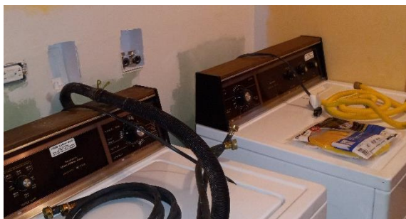
Install gas washer/dryer
