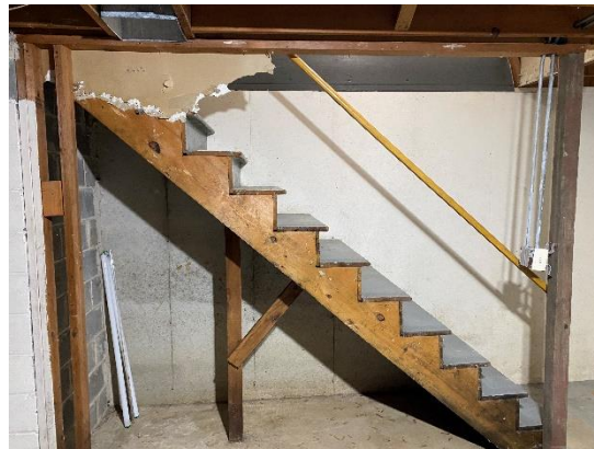
Finish Dry wall next to basement stairs and basement rooms
