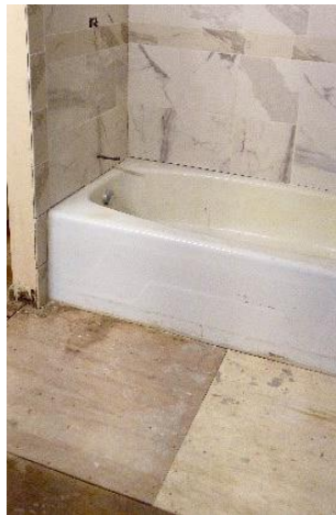
Install flooring in upstairs bathroom
